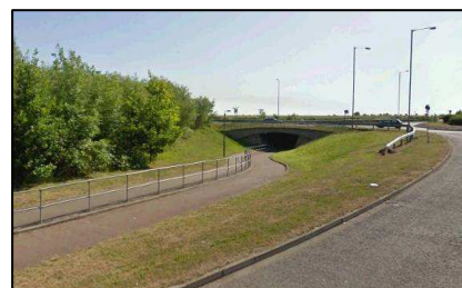
Pedestrian subway under the A507
