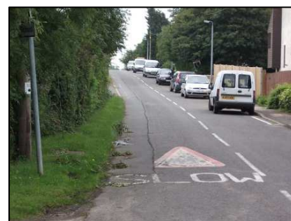
Lack of footpath on approach to Stondon Lower School
