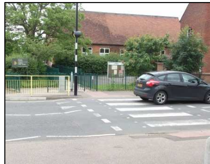
Raised zebra crossing outside Langford Lower School
